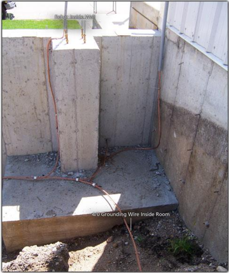
Figures 12 and 13. Room grounding wire connections to rebar inside wall
