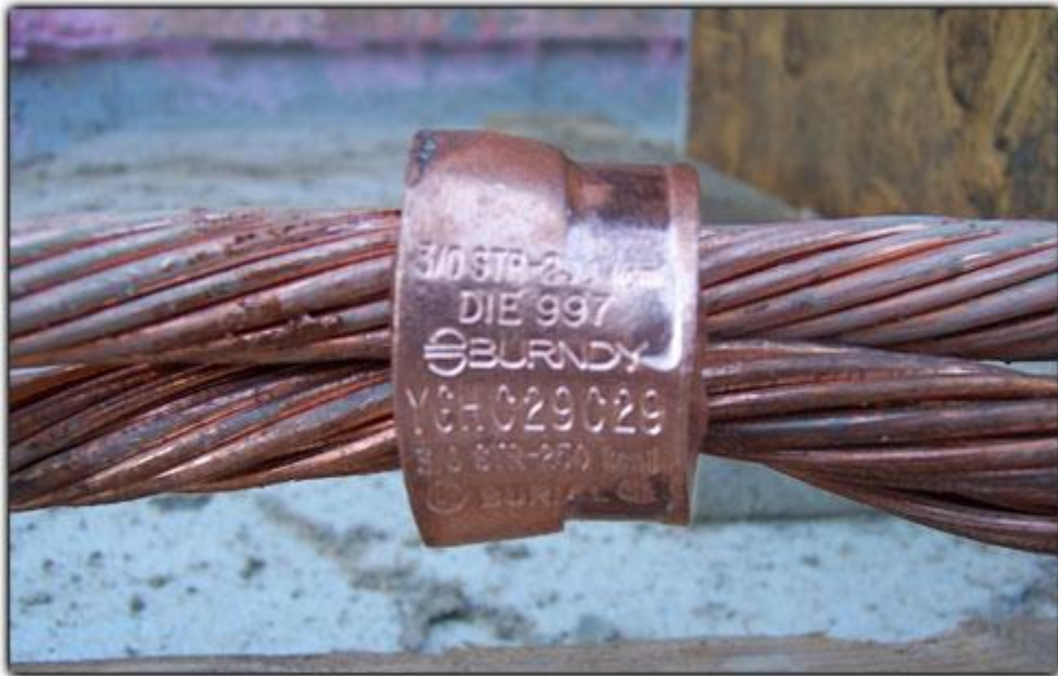
Figures 14 and 15. Properly crimped cable connections
