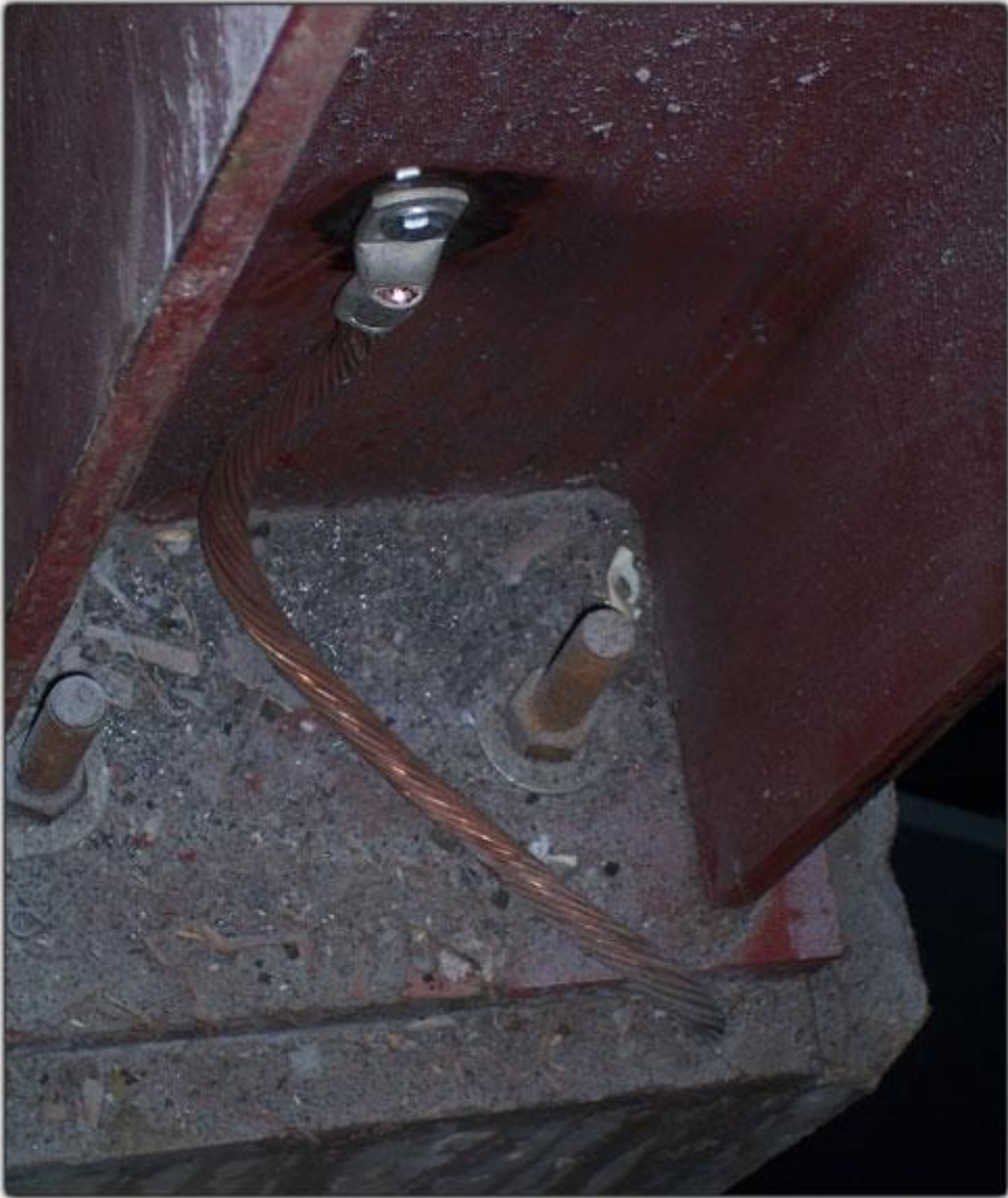
Figure 10. Proper ground connection to wall support
