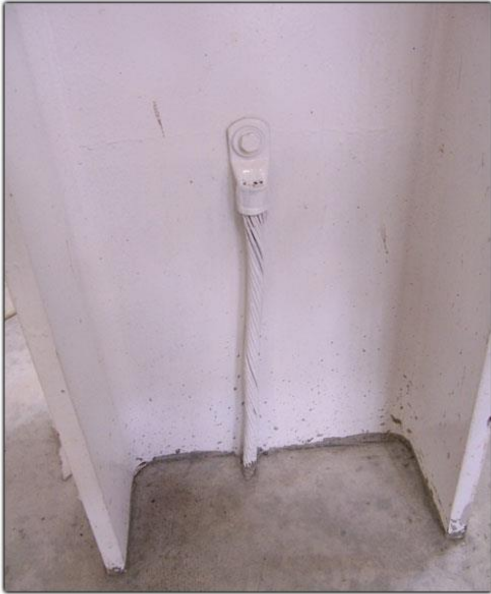
Figure 3. Ground connection made to metal beam before painting
